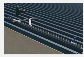
1. Measuring and predrilling the module field According to the design plan, the module field is measured on the roof. Then the trapezoidal sheet metal covering is pre-drilled using the TRITEC drilling jig.
