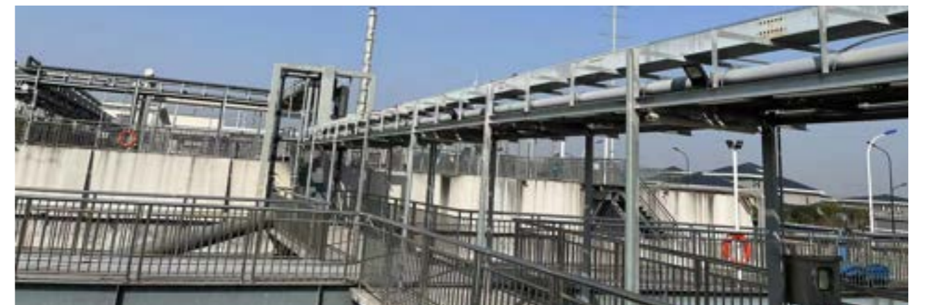
Aiko Solar Wastewater Treatment Station
